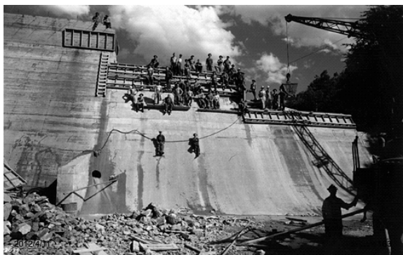
Workers at Big Ridge Dam Location : TN Agency : CCC, TVA
