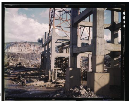
Early stage of construction work at the TVA's Douglas Dam, Tenn. 1942 June
